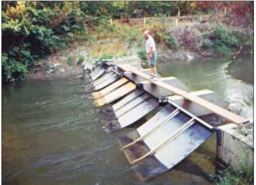
Pat Stevenson, environmental director with the Stillaguamish Tribe, checks out a flow control device that is helping fish in the Old Stillaguamish Channel. Photo: J. Shaw
